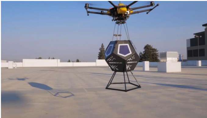
Drone Installation of Nokia LTE FCell
